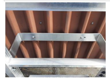
**22** Is the top of the ladder attached back to structure via a ladder bracket or to a structural platform within 300mm of the top rung? (NOTE: To be considered a structural attachment the ladder bracket must be secured back to either a concrete wall or structural steel beam or a steel/aluminium platform that is considered structural (Note: a standard platform or lead on kit is not considered structural) with a minimum thickness of 5mm, with a minimum of 3 x fixings no less than 12mm diameter)
