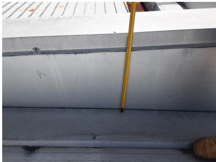
580mm parapet wall
