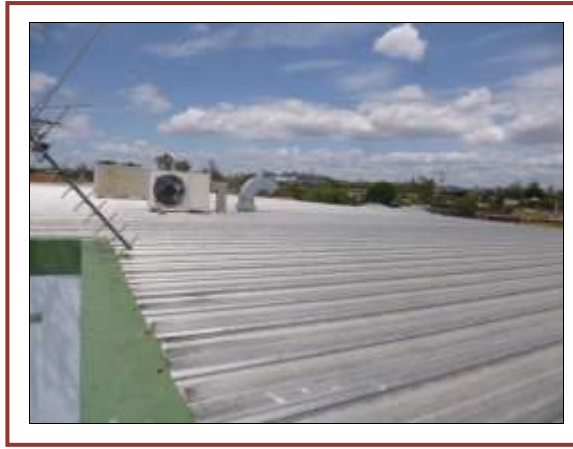
Photo #5 External Roof area No asbestos identified
