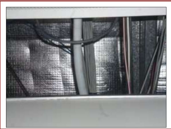
Photo #4 Internal Ceiling voids No asbestos identified
