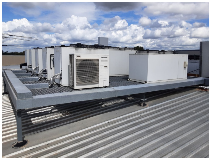
815mm drop off of plantdeck onto roof
