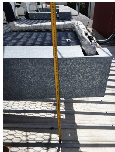
815mm drop off of plantdeck onto roof
