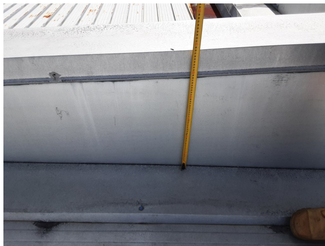
580mm parapet wall
